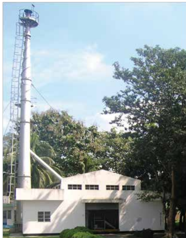
Effluent Treatment Plant (ETP) at GSK Chittagong Site.
