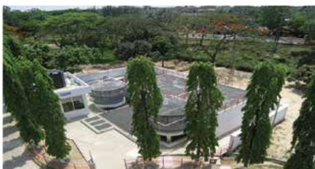
Effluent Treatment Plant (ETP) at GSK Chittagong Site.
